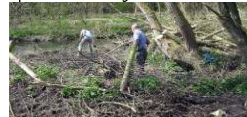
May 2008 Clearing Fiddlers Drain
